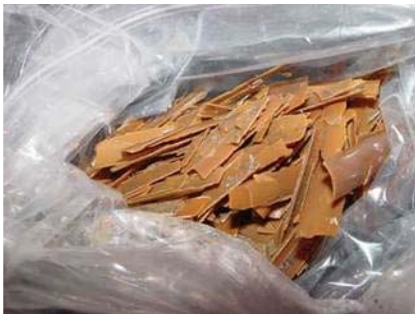
Pieces of the more than 8,000 pounds of calcium carbonate scale, pictured here, were removed from the tubes of STP's two condenser units. Photo courtesy of Conco Systems Inc.
