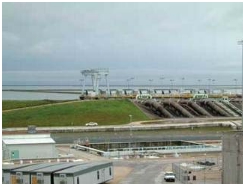
STP's 7,000 acre reservoir with inlet pipes to the condensers are pictured here. Photo courtesy of Conco Systems Inc.
