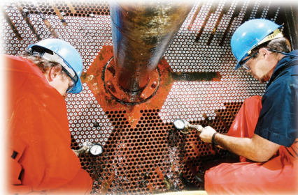
Technicians shooting Cal-busters to clean condenser at North Omaha Power Station. Photo: Courtesy of Conco Systems, Inc.
